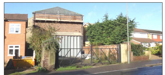
Thames Street warehouse, October 2014
